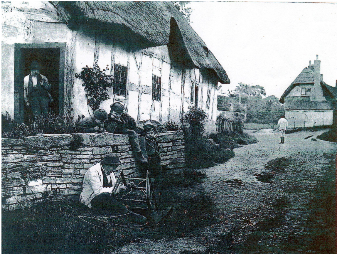
Running repairs outside Ten Penny Cottage, Boat Lane, Welford (1900s)
